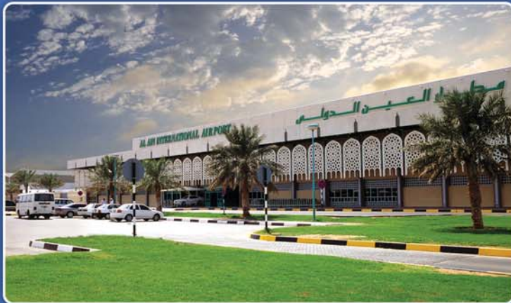
Al Ain International Airport, UAE
